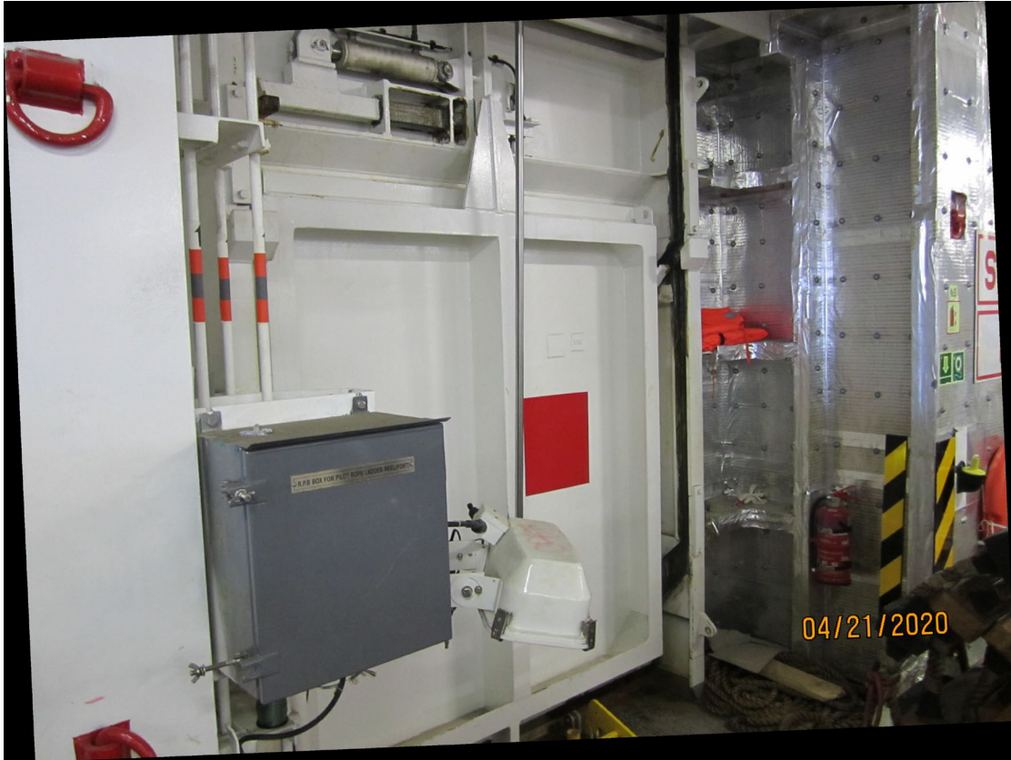
Figure 12. Photo of SILVER RAY Pilot Door closed taken from inside vessel by USCG
